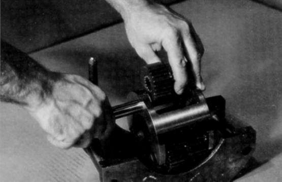
7. Following cluster gear, place one more thrust washer (3B) on planet shaft (3E) through opposite planet shaft hole in carrier housing (3A).
