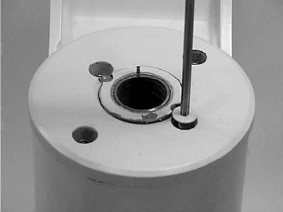
2. Using a 1/8" (3.18mm) drill bit, drill a hole in center of each lock pin to a depth of approximately 3/16" (4.76mm).
