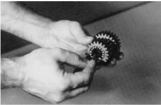
2. Place one spacer (3D) inside cluster gear (3F) so that it rests on top of the needle rollers.
