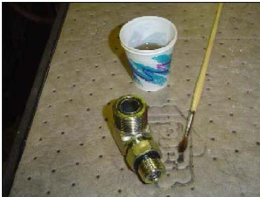
1. Hold fitting in one hand and dip brush into container with other hand. Remove excess hydraulic oil from brush so an even film of oil is applied to O-ring.
